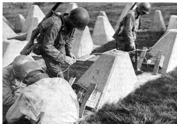
Figure 8: Improving the efficiency of Dragon's Teeth with explosive charges [19]
