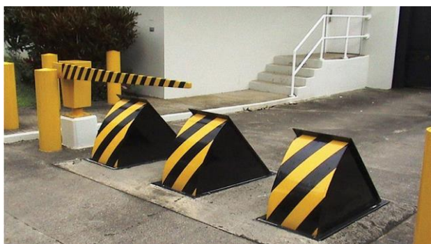
Figure 11: A mix of vehicle barriers in activated position [36]
